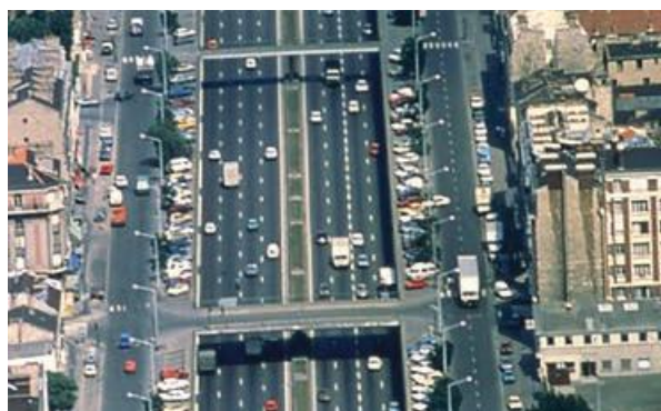
Photo 3 - Autoroute A1 avant requalification.
